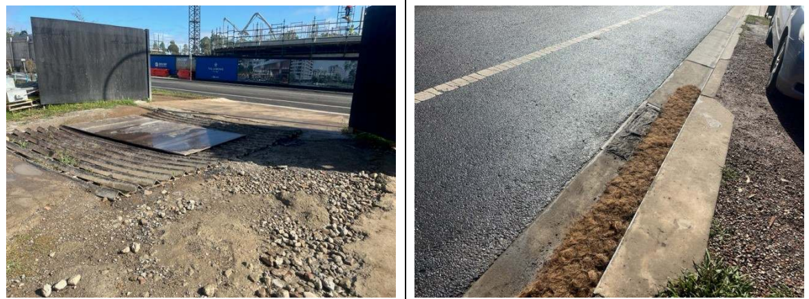
Photos 15 & 16: Stabilised site access and stormwater controls on Conferta Ave
