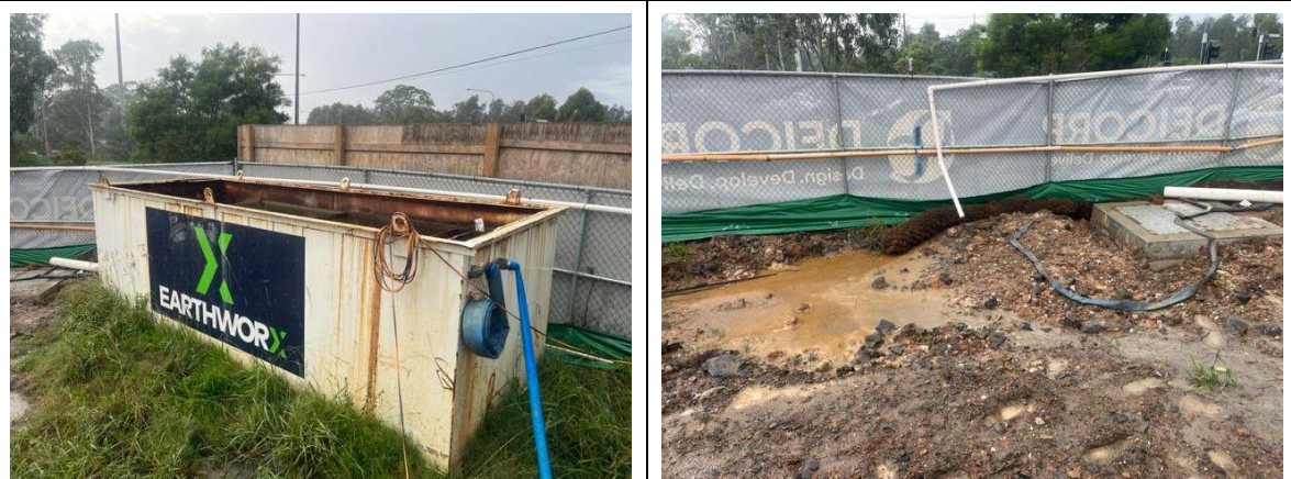
Photos 13 & 14: Sediment tank and discharge point to stormwater on Schofields Road
