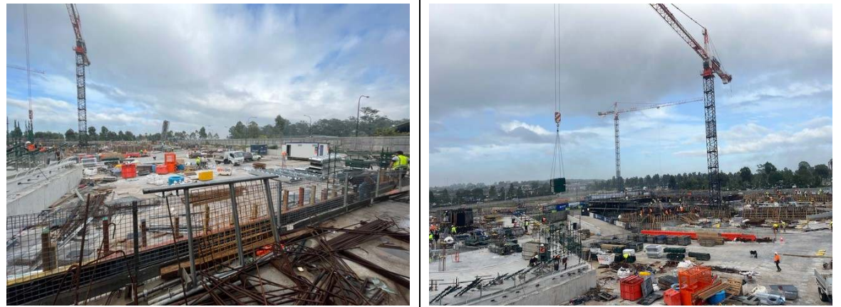
Photo 1: Site 1 – concreting, form reo pours and scaffolding
