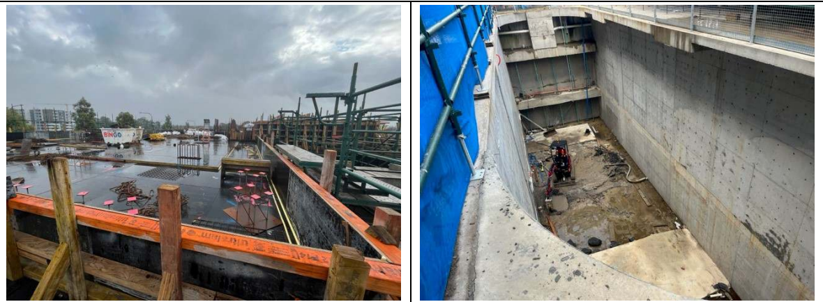
Photo 2: Site 1 – concreting, form reo pours and scaffolding
