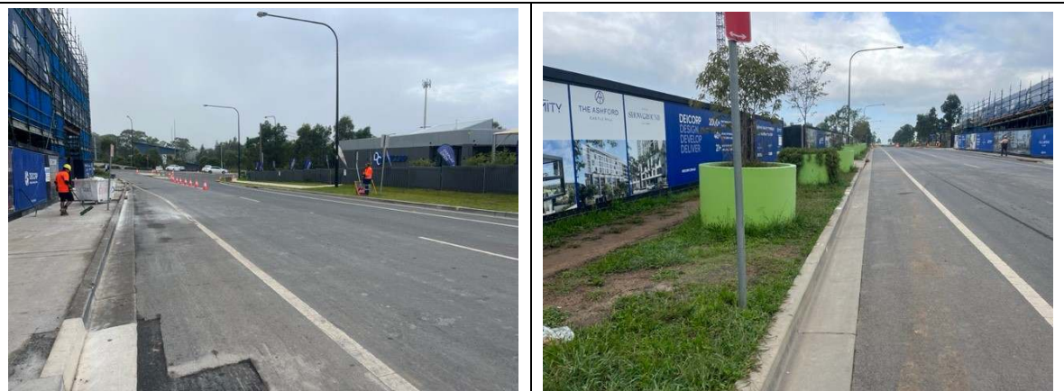
Photos 3&4: Conferta Ave – traffic control in place and use of regular sweeping evident
