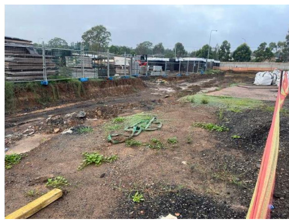
Photos 9&10: Site 2 – Central low point with discharge to sediment basin
